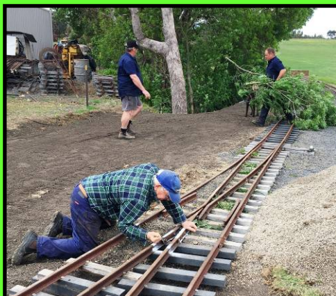
Relaying the Station Yard
