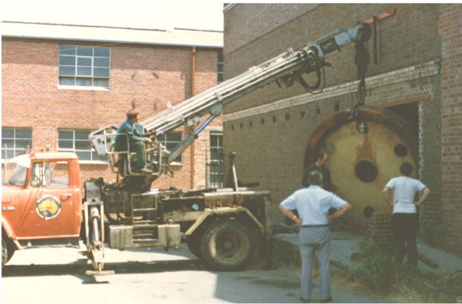
Loading the 7 tonne flywheel on the truck with Ray Gillett guiding (Ray Gillett)
